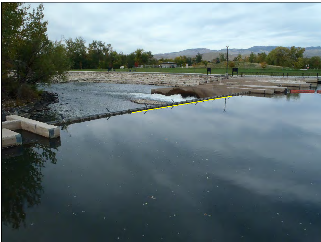
Photograph 1. Drop Structure 1 Gates 5 & 6 looking Downstream (October 2023).
