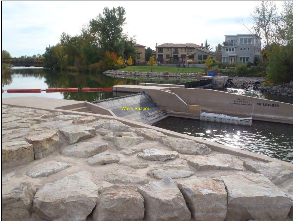
Photograph 5. Drop Structure 1 Wave Shaper looking Upstream (October 2023).
